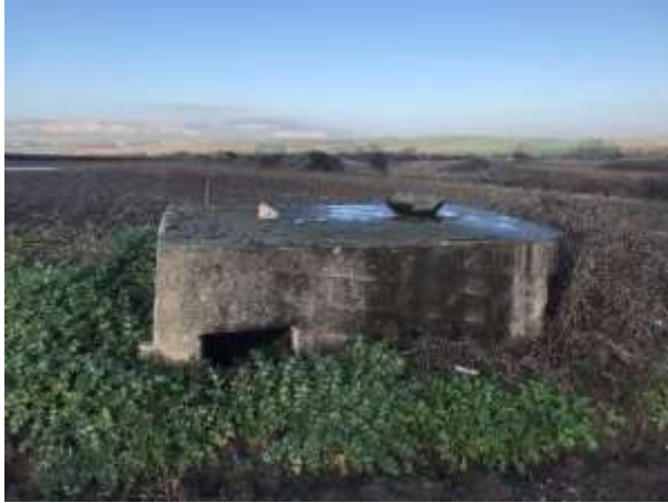
Photo 5: Historical Military Bunker – 293
