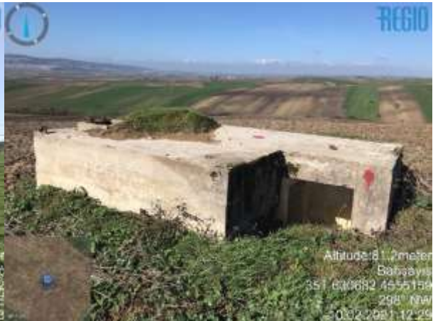
Photo 8: Historical Military Bunker – 296
